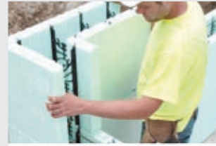
Stack forms & create openings
