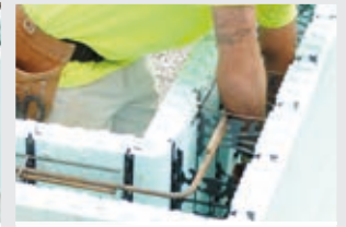
Place rebar in the walls
