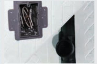
Install electrical, plumbing & roof
